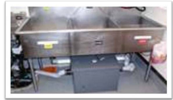
Hydromechanical Interceptor (Under Sink Grease Trap)
