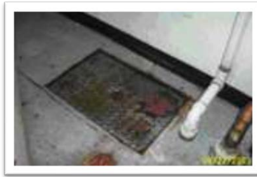
Hydromechanical Interceptor (In-Floor Grease Trap)
